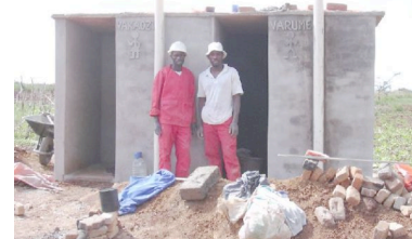
Building a Blair toilet
